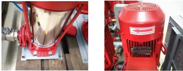
Figure 8.2 Booster rotation direction
