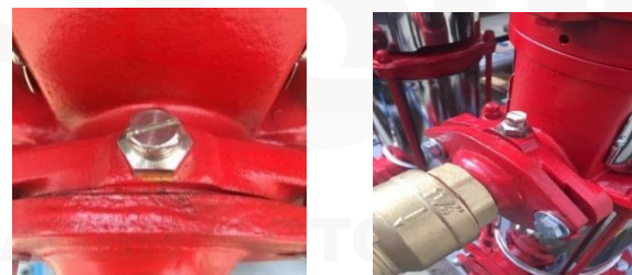
Figure 8.1. Booster air plug
